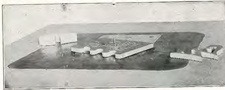
Figure 13—The Saw Table mounted flush with the bench top
